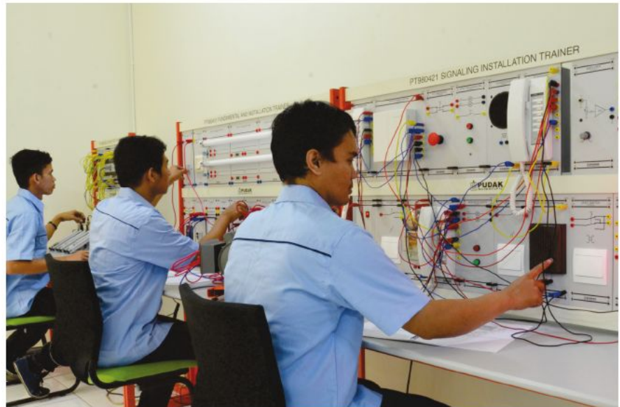
Training Panel System in Lab. Setting
